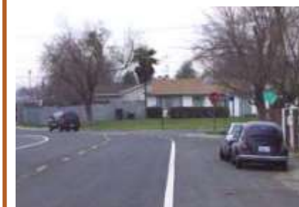
Edge lines are a cheap, effective way to visually narrow a street and reduce vehicle speeds. Edge lines also can create a shoulder, parking area, or bike lanes.
