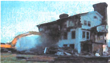
Demolishing houses can make room for redevelopment and remove nuisances. But demolition also removes older, historic buildings and can create voids.
