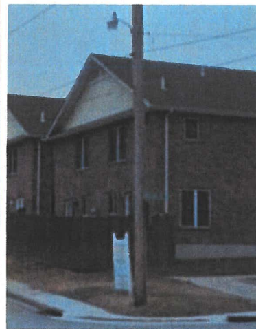
Streetlights are generally located at street intersections. A few additional streetlights may be needed in the neighborhood. Coordination may be needed due to existing trees and utilities.
